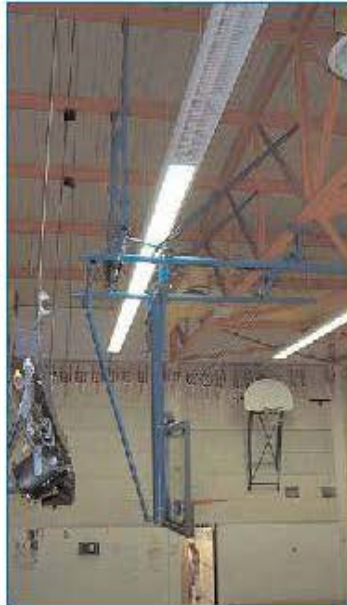
Custom Ceiling Bracing for Single Mast Unit 2 different beam heights, avoiding lights. Installed at Woodbridge College
